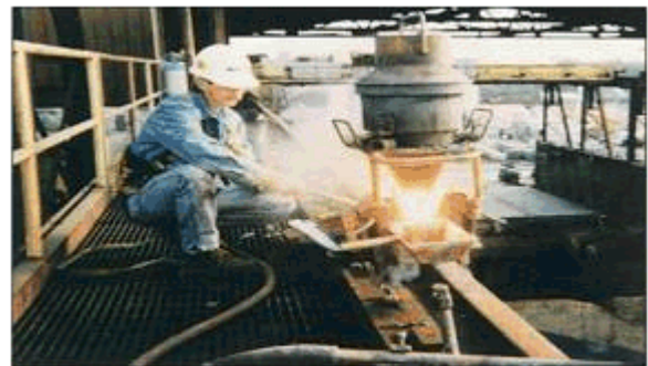
Thermal Rail Welding
