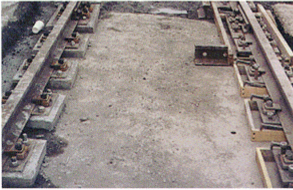
Fig. 5 — Intermittent soleplate rail system.
